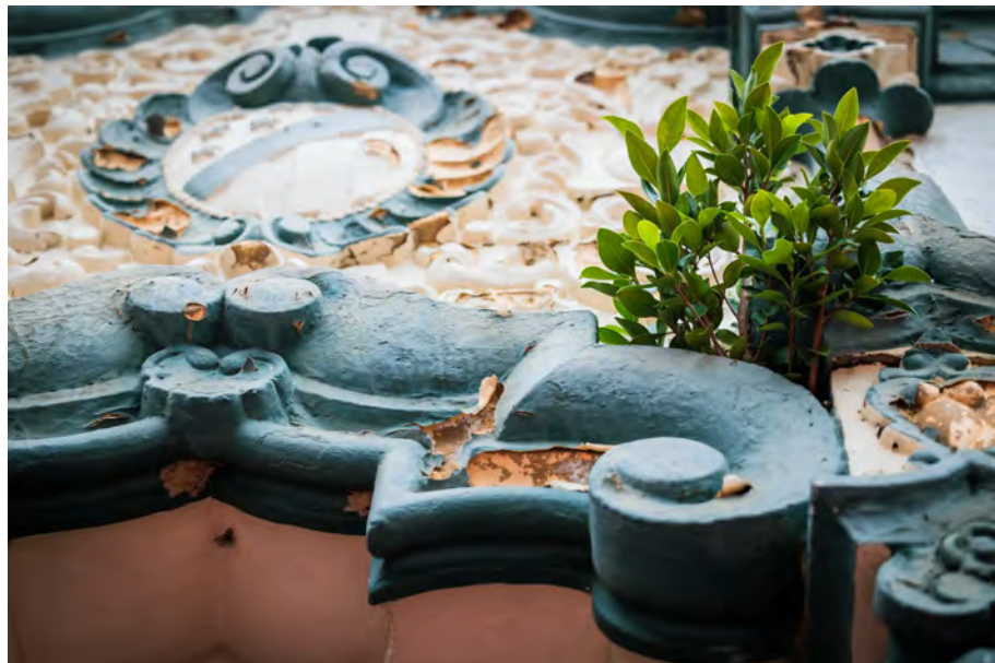
Foliage grows out of the some of moluding on the facade of the Recreation Park Band Shell. (Richard H. Grant | Signal Tribune)
