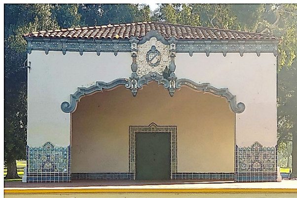
Stage Side Building
