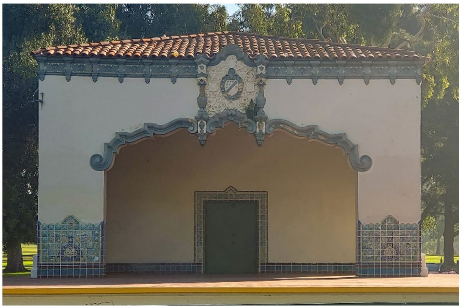
Stage Side Building
